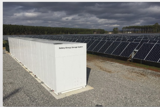
Redstone Arsenal, Alabama: 10 megawatt (MW) alternating current solar project with Army's first privately funded, commercially available battery storage solution
